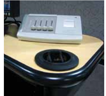
Diffusers Diffusers supply filtered air to the desktop and are adjustable to direct airflow.
