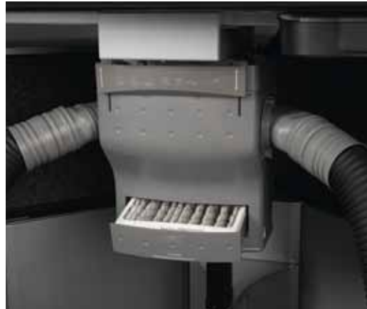
Electronics unit Electronics unit mounts to the underside of a surface and includes a particle filter that is easily serviced.
