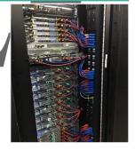
as show would allow for standardization on shorter (18") cords and eliminate cable bundling and reduce all airflow impact to negligible impact. This may have operational cost benefit and reduced cooling needs.
